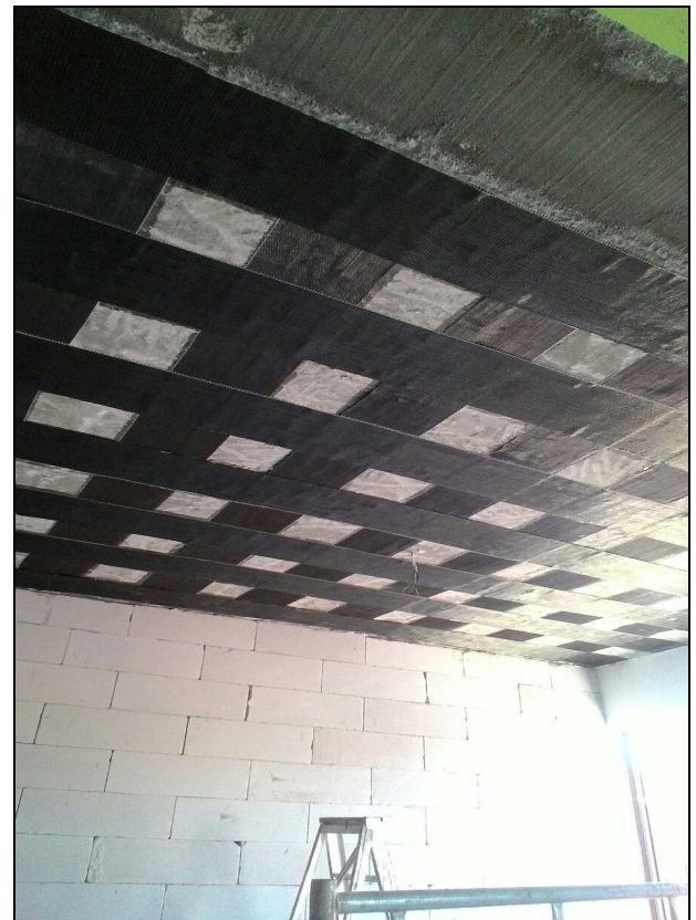
Build Wrap AAA 300, apply on Slab
