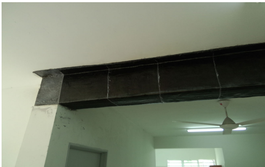
Completed Apply of Build Wrap AAA 300
