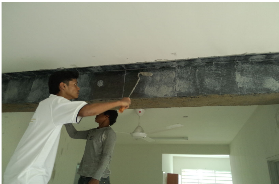
Surfaces Preparation, Apply of Epoxy Primer
