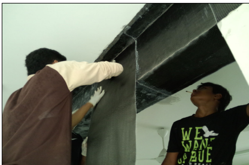
Apply of Build Wrap AAA 300 on Beam
