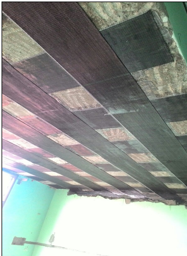
Build Wrap AAA 300, apply on Slab
